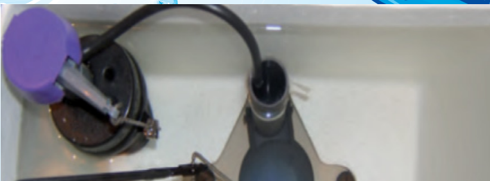
Building "A" is 7 years old and had a JUDO Profimat water strainer installed when constructed. Sediment and rust free toilet tank and aerator.
